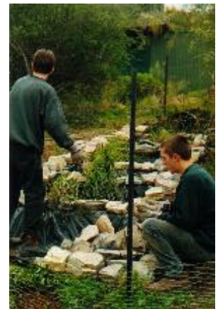
Landscaping projects around the home – building a greywater system.
