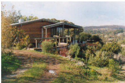
The house that Robin, Beverley, April and Roger built.
